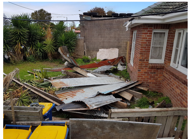
Storm debris that blew from a neighbouring (non-HNZ property) into one of our properties
